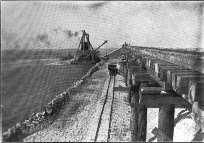
APPROACH TO THE LONG KEY VIADUCT IN PROCESS OF CONSTRUCTION.
