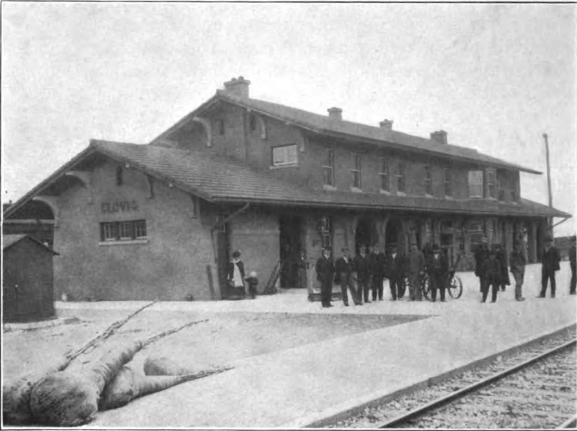
STATION AT CLOVIS, N. M., ON THE BELEN CUT-OFF. Showing the type of fireproof construction and the standards set in developing even a new country. Clovis is a division point on the new Santa Fe 0.6 per-cent-grade line for transcontinental heavy through freight. The saplings on the platform are to be planted in this new town.
