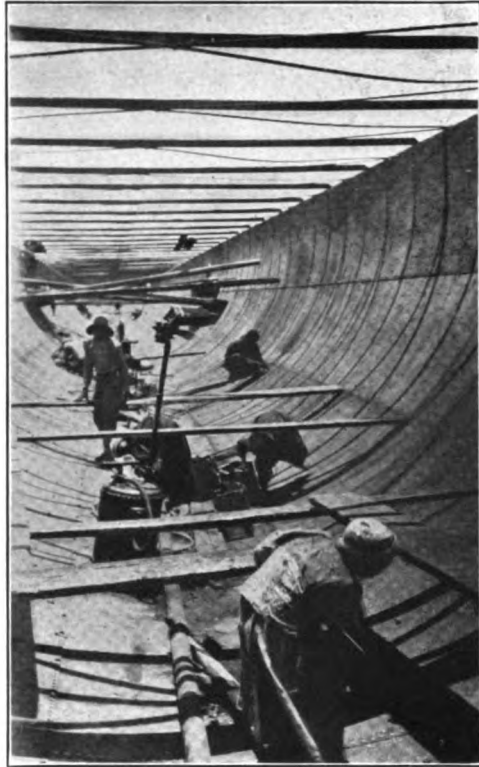
RIVETERS AT WORK IN THE INTERIOR OF THE STEEL CANAL.
