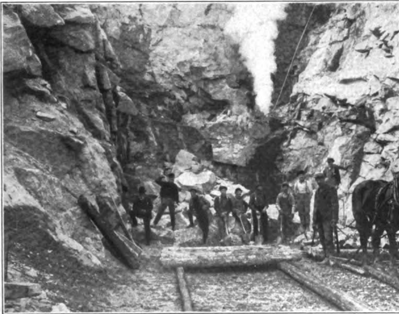
THE FACE OF A 50-FOOT CUT.
