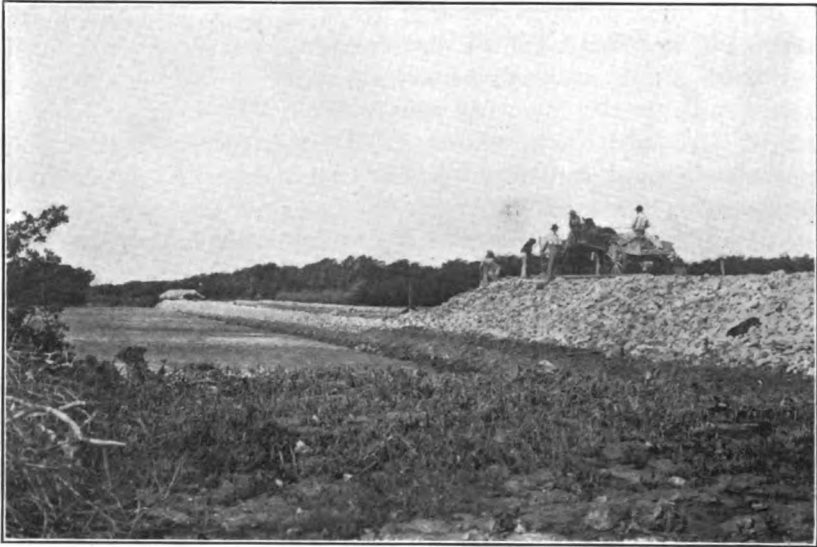
ROCK FILL AT PULL-AND-BE-DAMNED CREEK.
