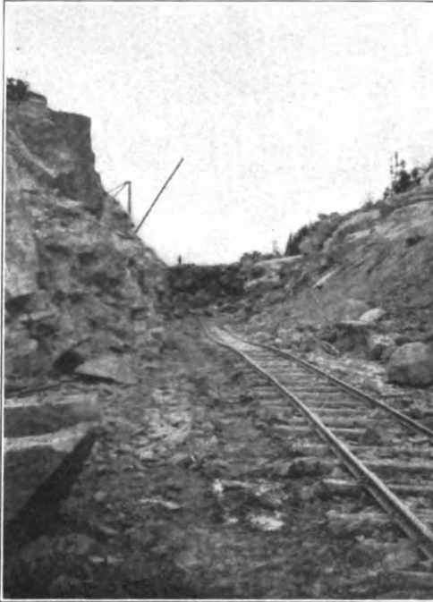
A ROCK CUT NEARLY FINISHED.
