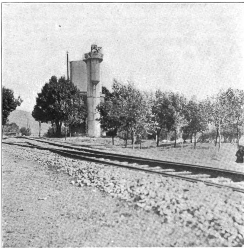
AN UNUSUALLY FINE TANK ON THE EST-ALGÉRIEN RAILWAY, AT EL GUERRAH.
