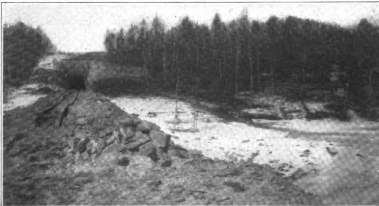
ROCK FILL ACROSS A BAY OF LAKE ENA, SHOWING SUBSIDENCE.
