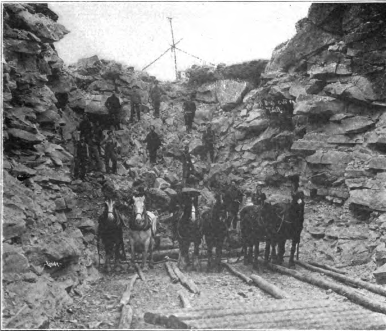
MUCKING OUT FROM A HEAVY CUT.
