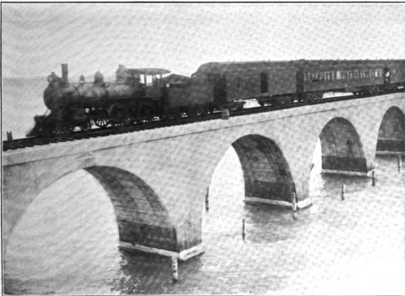
THE COMPLETED VIADUCT.
