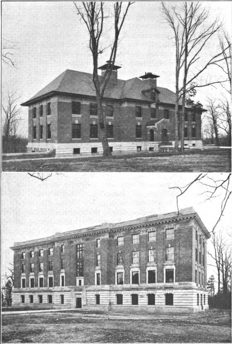
THE MECHANICAL LABORATORY AND POWER PLANT (ABOVE) AND THE PHYSICAL LABORATORY, NATIONAL BUREAU OF STANDARDS.
