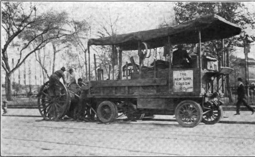
ELECTRIC 5-TON TRUCK WITH POWER WINCH FOR HAULING CABLE THROUGH CONDUITS.
