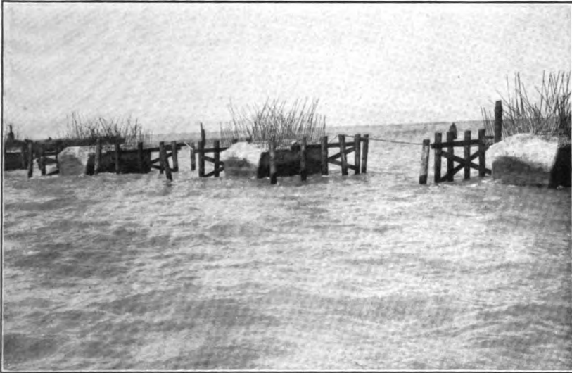
FINISHED PIERS OF THE LONG KEY VIADUCT.
