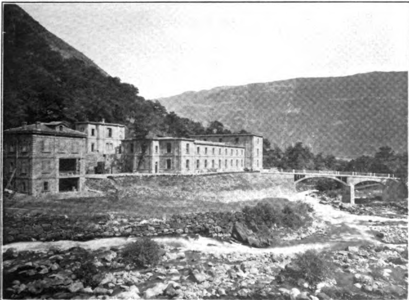
FIG. 12. BRIDGE AT THE PIATTAMALA STATION.
