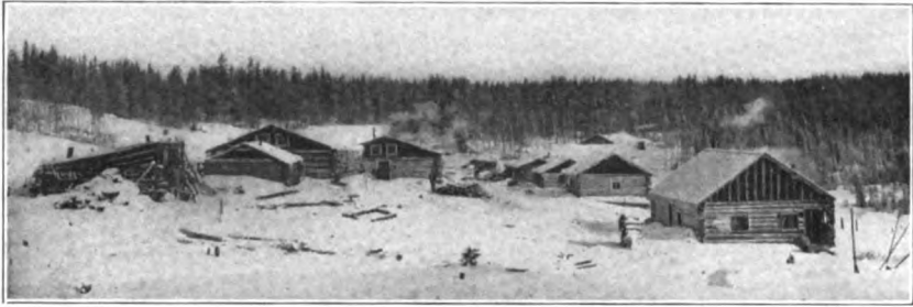
A CHARACTERISTIC RAILWAY CONSTRUCTION CAMP; CHAMBERS' NO. 5.
