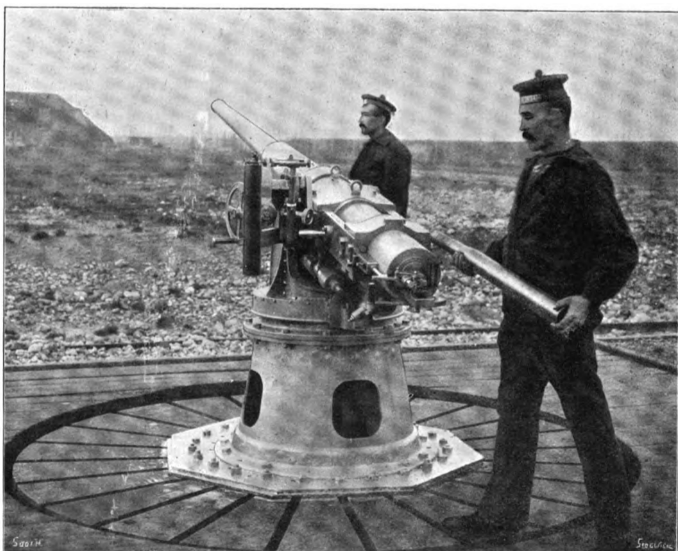
FIG. 575. MOUNTING FOR 57-MILLIMETRE QUICK-FIRING GUN.
