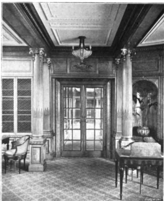
FIG. 74. VIEW FROM LIBRARY, LOOKING TOWARDS GRAND ENTRANCE AND LOUNGE.
