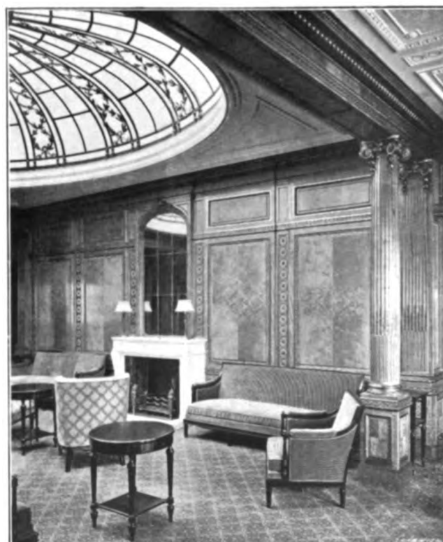
FIG. 75. FIREPLACE IN LIBRARY, WITH SYCAMORE PANNELING.
