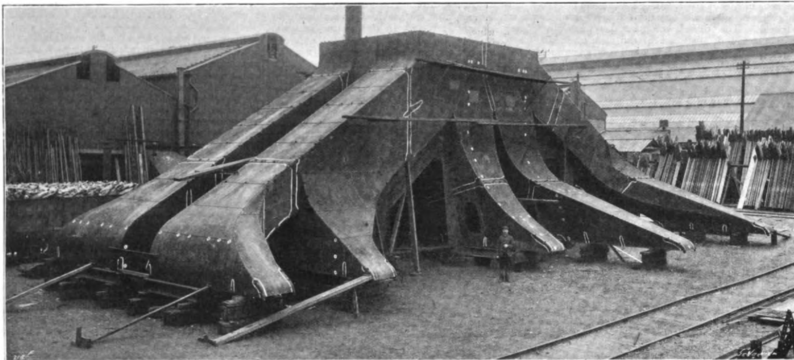
FIG. 172. UPTAKE FOR SIX BOILERS.
