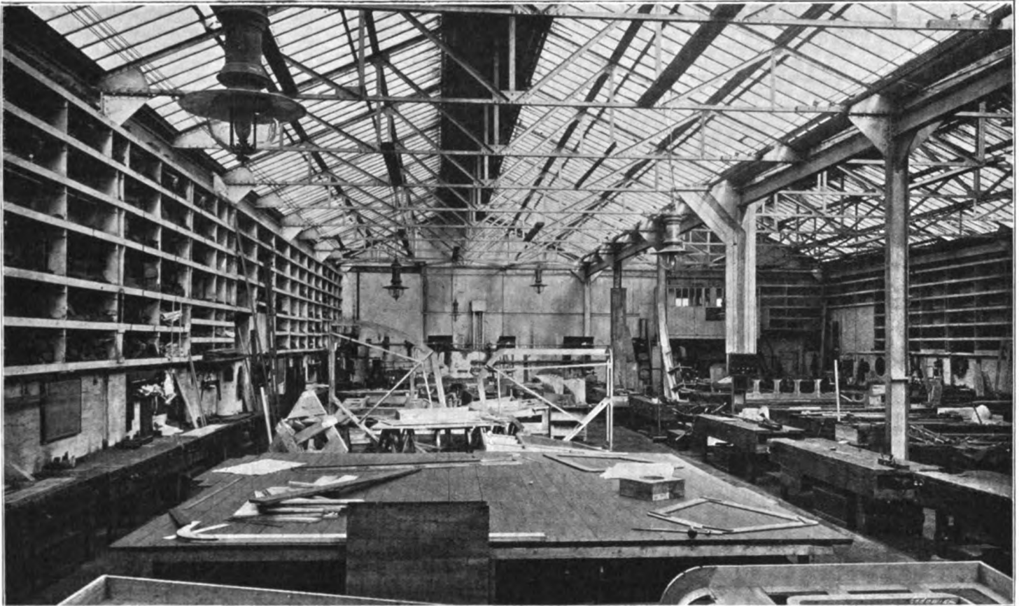
FIG. 113. THE PATTERN SHOP AT THE WALLSEND ENGINEERING WORKS.
