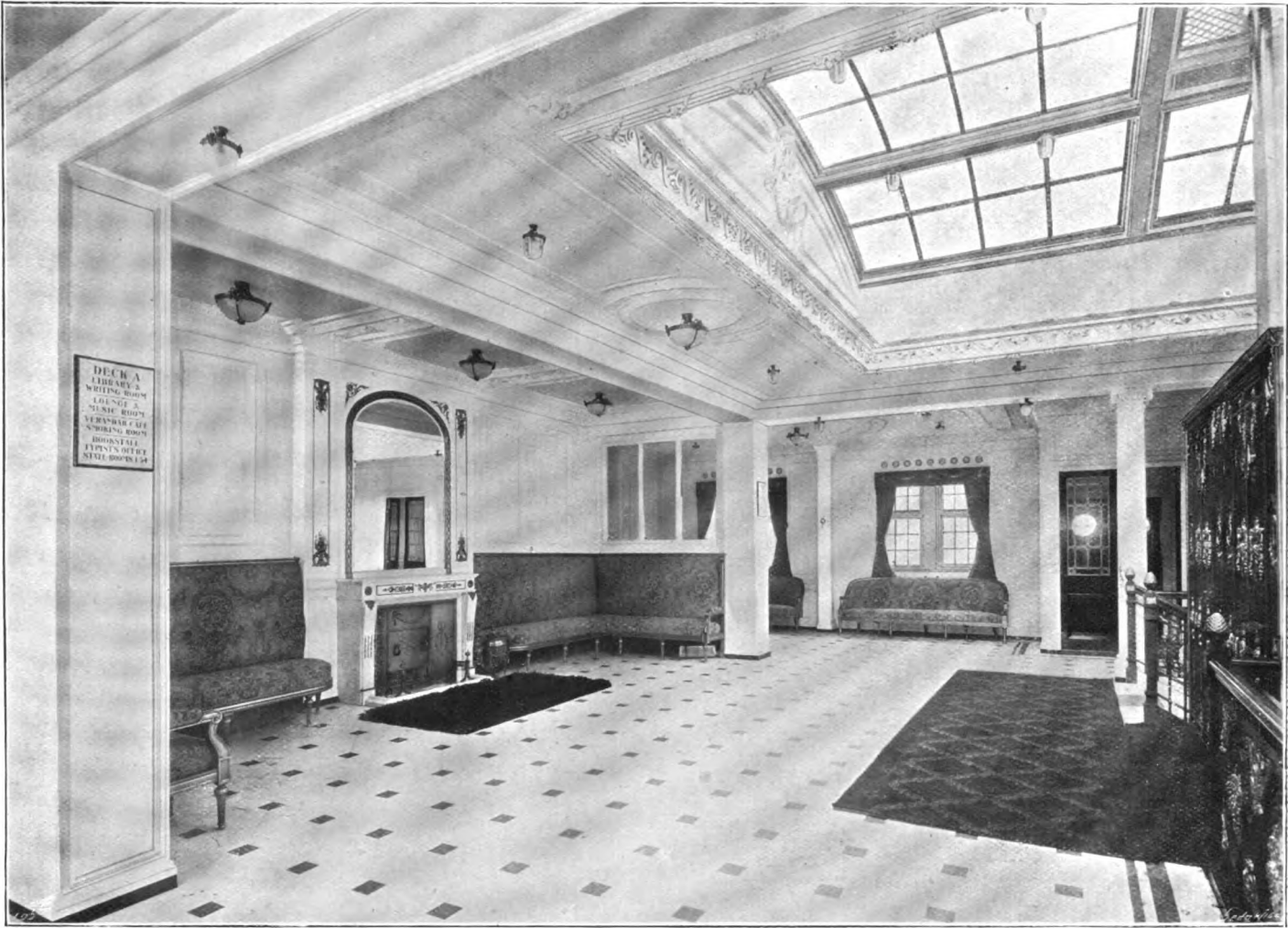
FIG. 10. THE ENTRANCE HALL ON THE SHELTER-DECK, WITH HOISTS.
